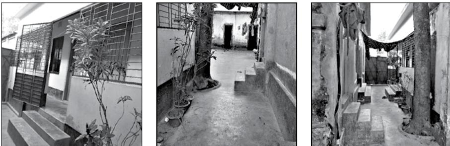
**Figure-24:** High plinth of the new constructed two buildings of the selected homestead compare to the previous buildings of that homestead. (Source: Author's photographs)
