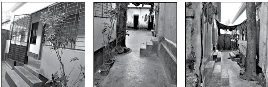
**Figure-24:** High plinth of the new constructed two buildings of the selected homestead compare to the previous buildings of that homestead. (Source: Author's photographs)
