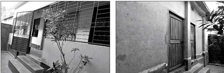
**Figure-13:** High plinth in the newly constructed buildings. (Source: Author's photographs)
