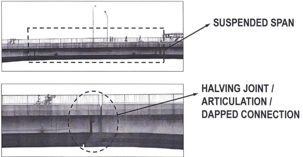
Fig.19: Articulation/ Halving joint
