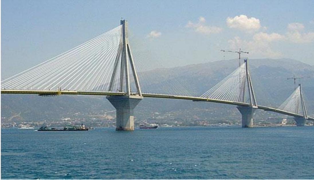
Fig.4: Cable-stayed Bridge – *Rion Antirion Bridge, Greece* (Source :online)
