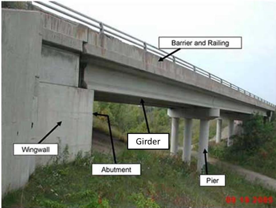
Fig. 8: Different components of a Bridge
