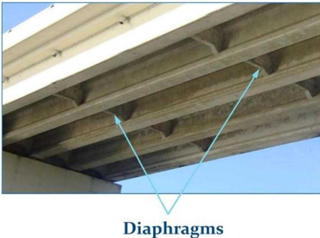
Fig. 23: Diaphragm or cross girder of Sebastian Intel Bridge, Florida, USA
