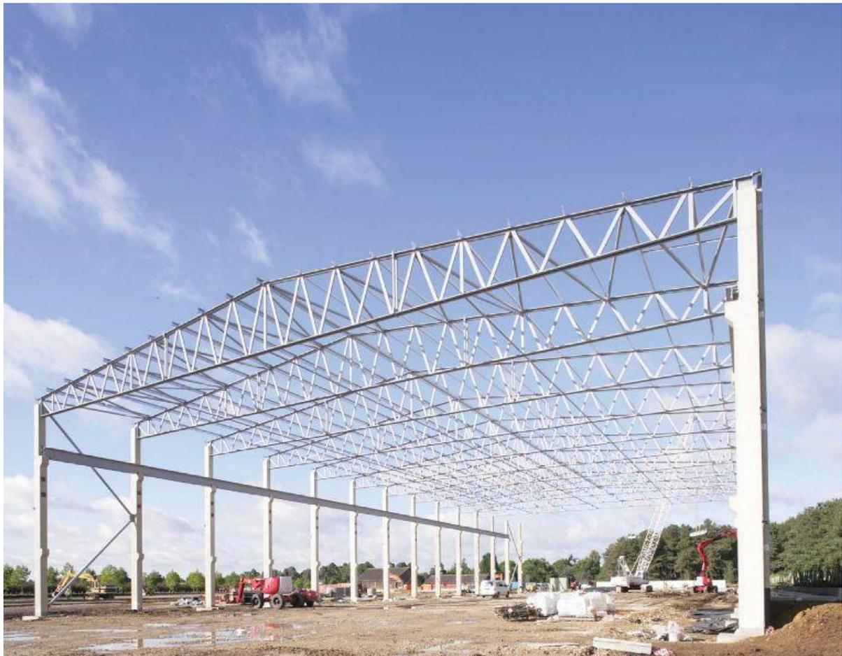
**Figure 2.1: Truss Structure**
