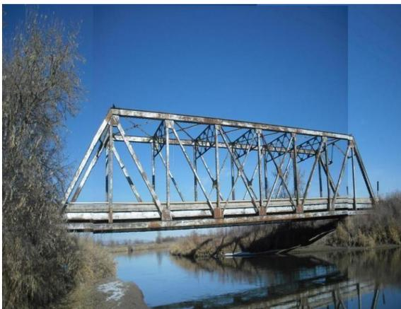
**Figure 1.2(a): Truss bridge (Trenton
