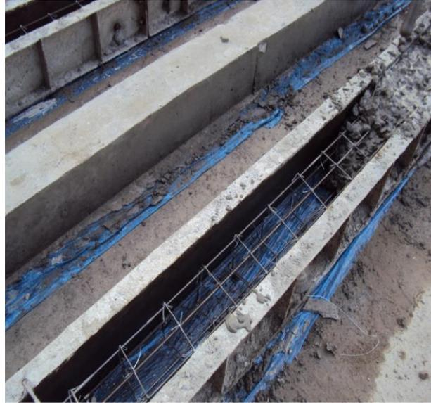
**Fig. 2.41** Placing of shuttering (step 03)
