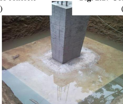
**Fig. 2.18** Curing of concrete
