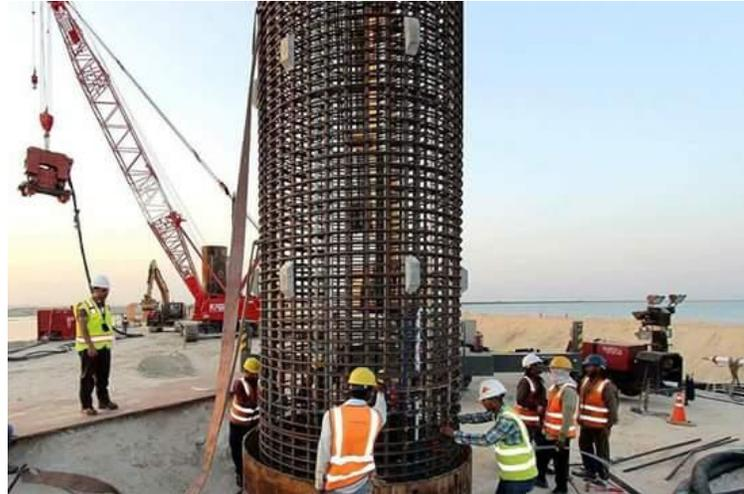
**Fig. 2.53** Welding of casings
