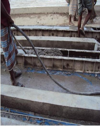
**Fig. 2.44** Compaction of concrete
