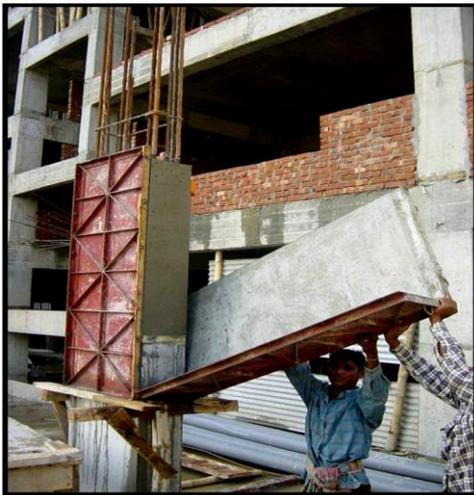
**Fig. 3.12** Removal of shuttering
