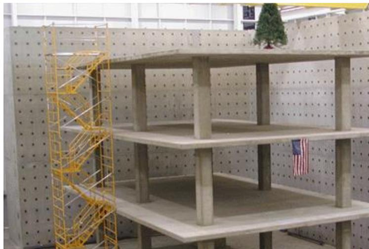
**Fig. 1.13** Flat plate structure
