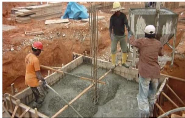
**Fig. 2.17** Compaction of concrete
