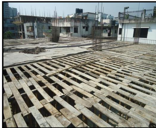
**Fig. 3.26** Timber formwork
