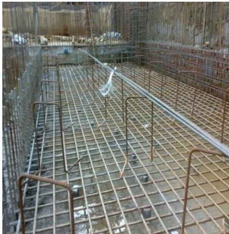
**Fig. 2.31** Reinforcement placing
