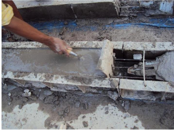
**Fig. 2.45** Leveling top surface
