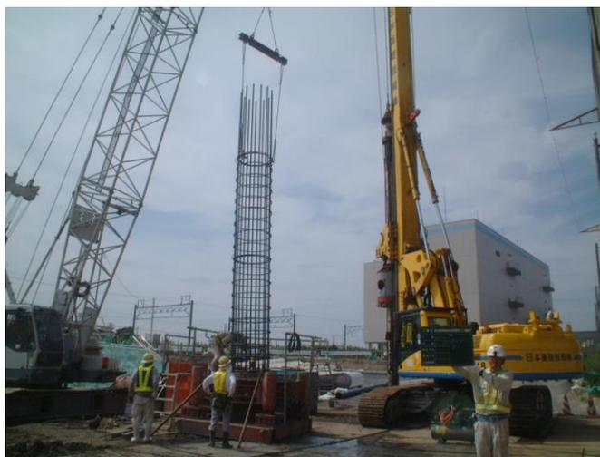
**Fig. 2.52** Reinforcement casing placing
