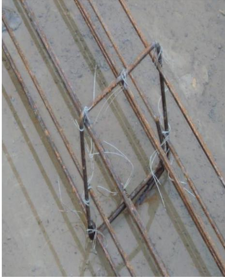
**Fig. 2.40** Reinforcement casing construction (step 01)
