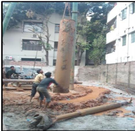
**Fig. 2.5** Temporary casing placement
