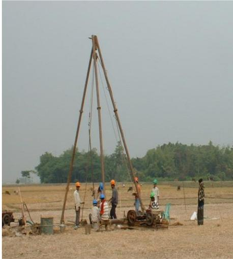
**Fig. 2.3** Placement of pipe derrick
