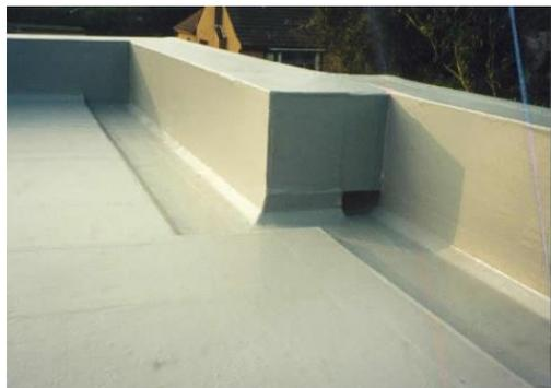
**Fig. 8.1** Parapet
