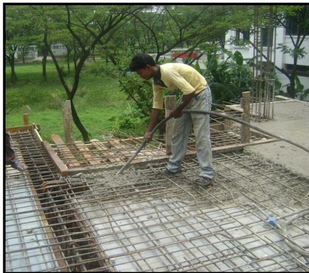
**Fig. 3.23** Monolithic casting of beam and slab
