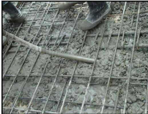
**Fig. 3.31** Compaction
