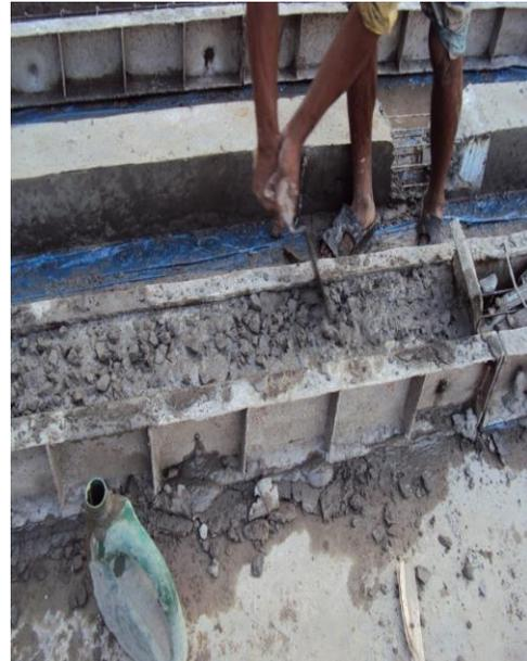
**Fig. 2.43** Casting of concrete (step 05)
