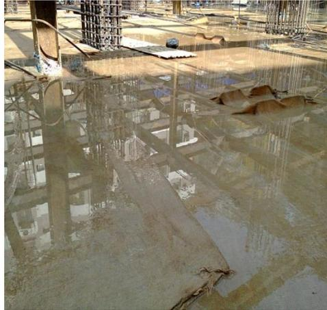
**Fig. 2.33** Concrete curing
