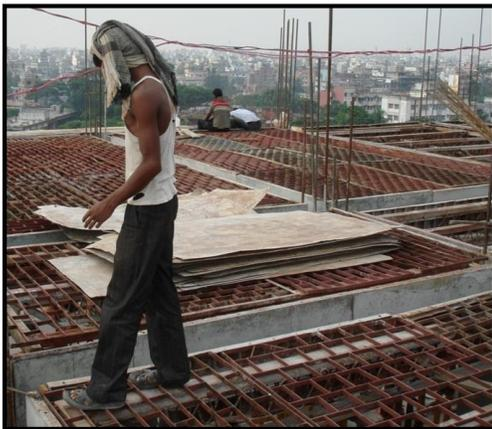
**Fig. 3.25** Steel formwork
