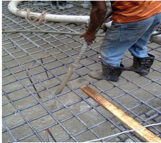
**Fig. 2.34** Concrete compaction
