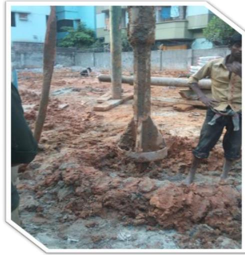
**Fig. 2.4** Centering and Placing of Augur
