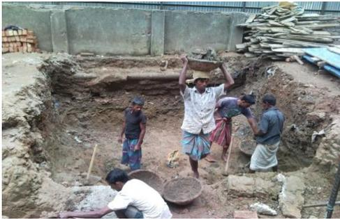
**Fig. 2.10** Excavation of trench
