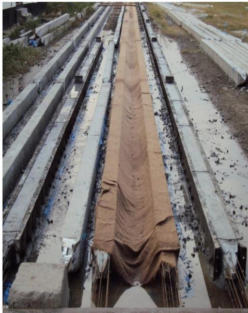
**Fig. 2.46** Curing of concrete
