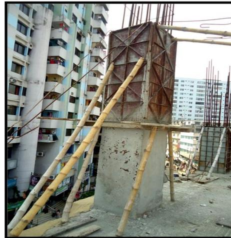
**Fig. 3.10** Concrete Casting in two lifts
