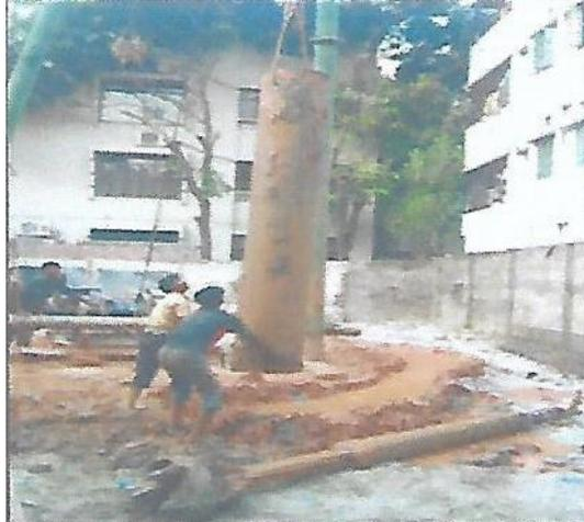
**Fig. 2.49** Temporary Casing insertion
