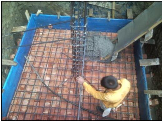
**Fig. 2.16** Casting of concrete
