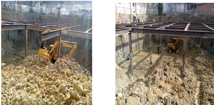
**Fig. 2.22** Soil Excavation
