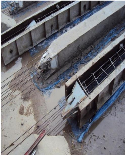
**Fig. 2.42** Inserting steel cap (step 04)
