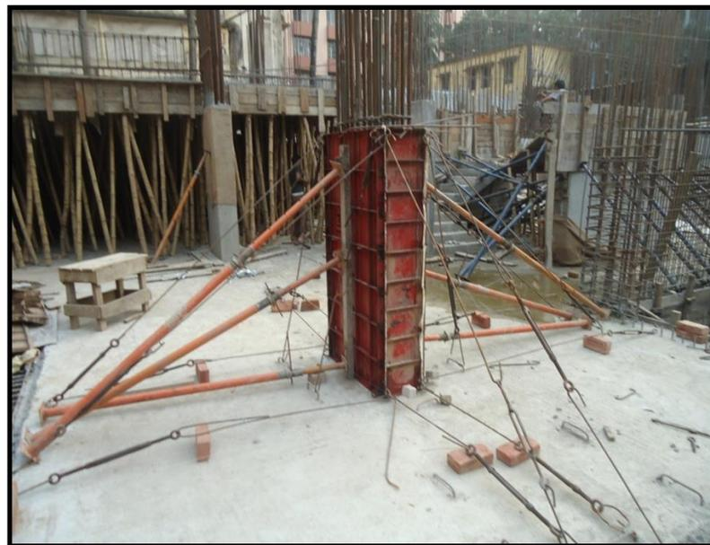
**Fig. 3.7** Steel shuttering
