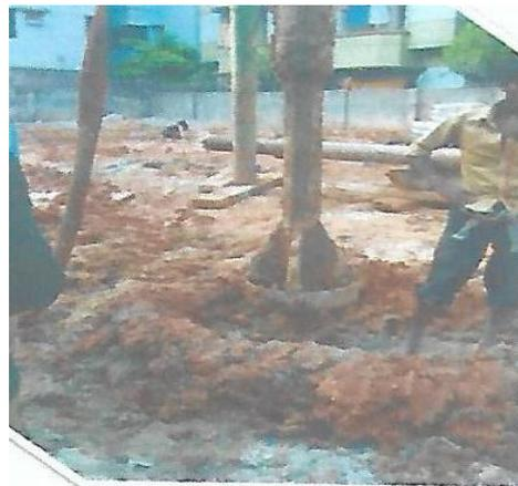
**Fig. 2.48** Centering and Placing of Auger
