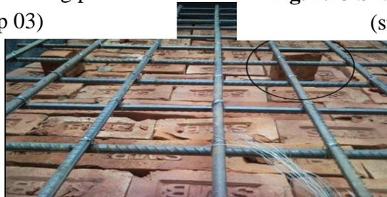
**Fig. 2.14** C.C. block placement
