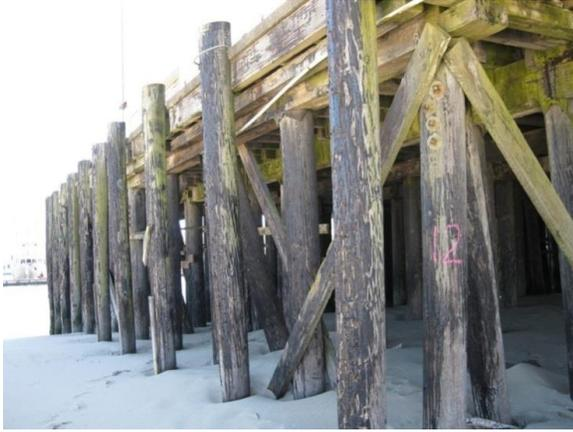
**Fig. 2.37** Timber pile
