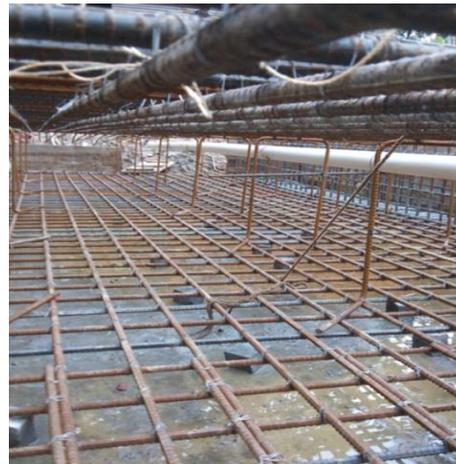
**Fig. 2.32** Reinforcement placing
