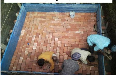
**Fig. 2.12** Brick flat soling placement
