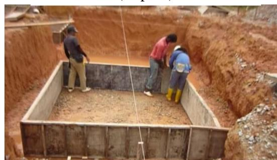
**Fig. 2.13** Shuttering placement
