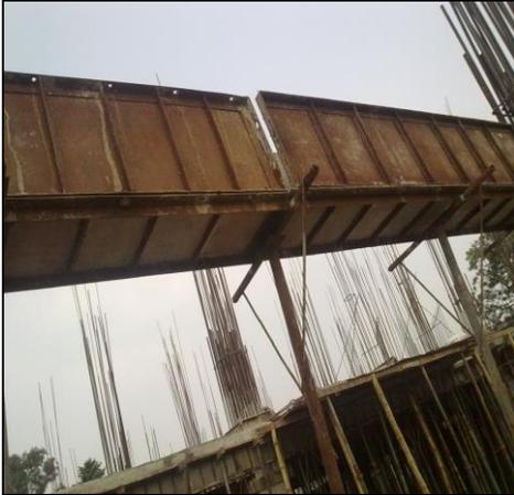
**Fig. 3.14** Steel formwork
