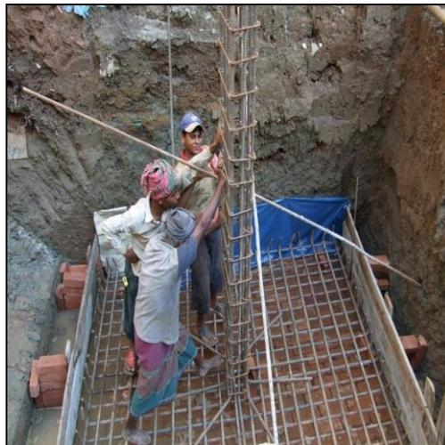
**Fig. 3.1** Placing column reinforcement
