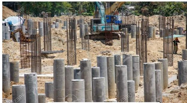
**Fig. 2.39** Concrete pile
