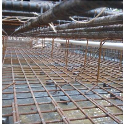
**Fig. 2.30** Placing CC block
